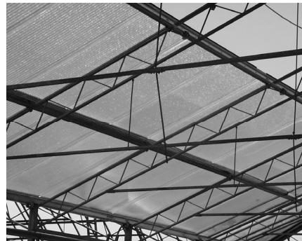
Fig. 7b. Detail of the roof construction of the wide span greenhouse in Assendelft.
