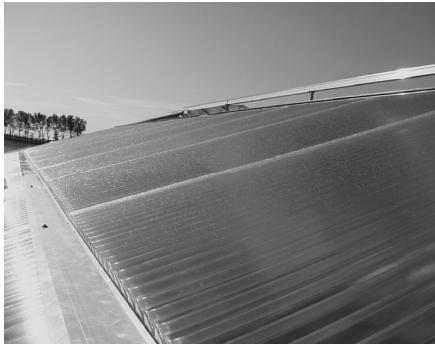
Fig. 7a. First wide span greenhouse with extruded zigzag in Assendelft (Netherlands).
