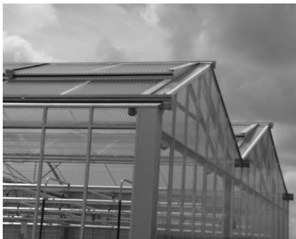
Fig. 6a. First greenhouse with Extruded zigzag sheets: Lexan® Zig Zag™ in Elst (Netherlands).
