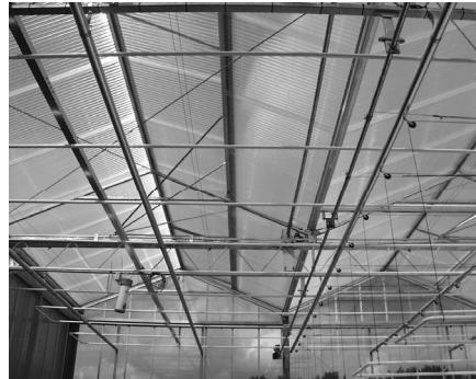
Fig. 6b. Detail of the roof construction with the extruded ZigZag sheets.
